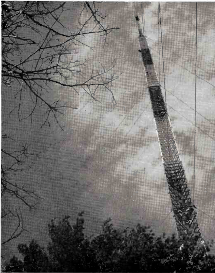
above—WBZ-TV's new Ideco tower at Boston, 1,199 feet above ground (1,349 feet Mean Sea Level). right—Slot antenna will side-mount directly beneath WBZ-TV's present antenna. The super-gain antenna will bolt into the bottom section of the narrow tower top.
